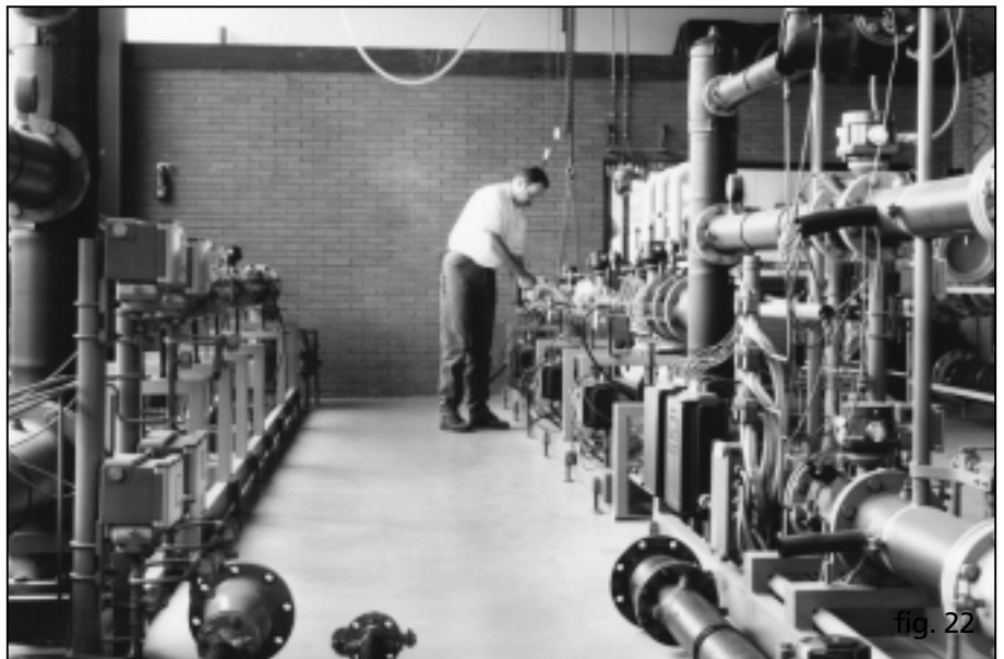
fig. 22 Instromet Natural Gas High Pressure Calibration Facility in Utrecht, The Netherlands
